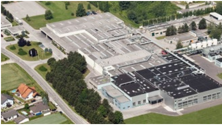
Bio Pharma Plant #1
